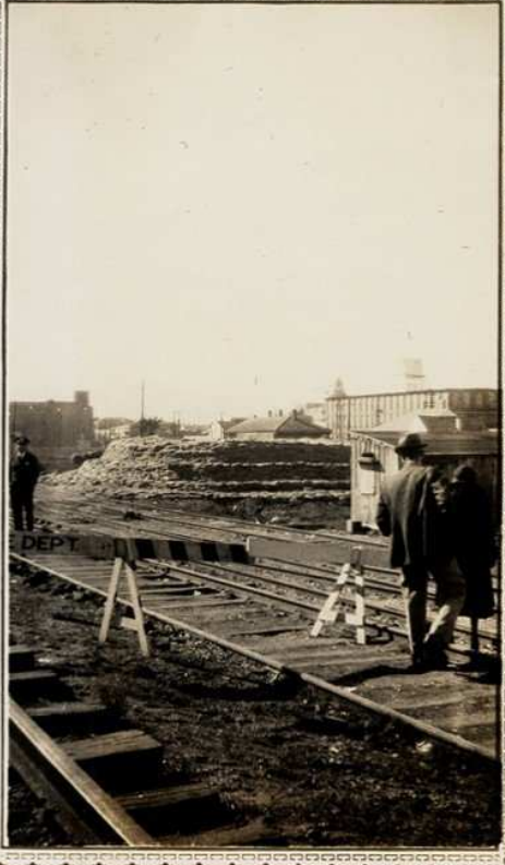
Sand Bags on levee march 1937
