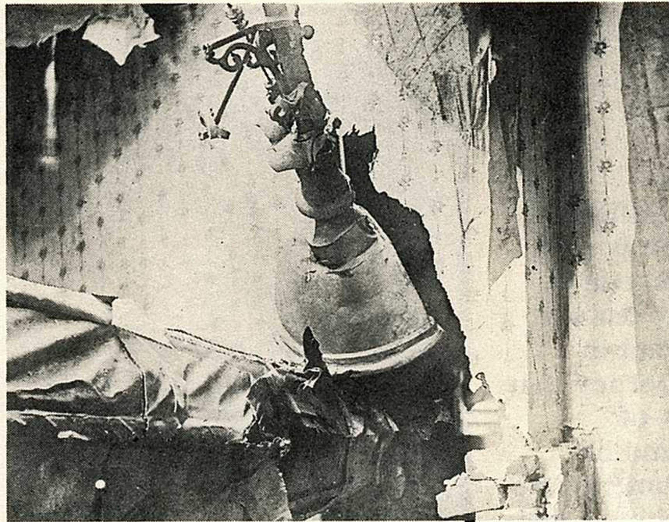
St. Paul's steeple crashed into the third house from the church. It fell across the bed and the top landed in the fireplace. The school building & adjoining cottage were completely demolished.
