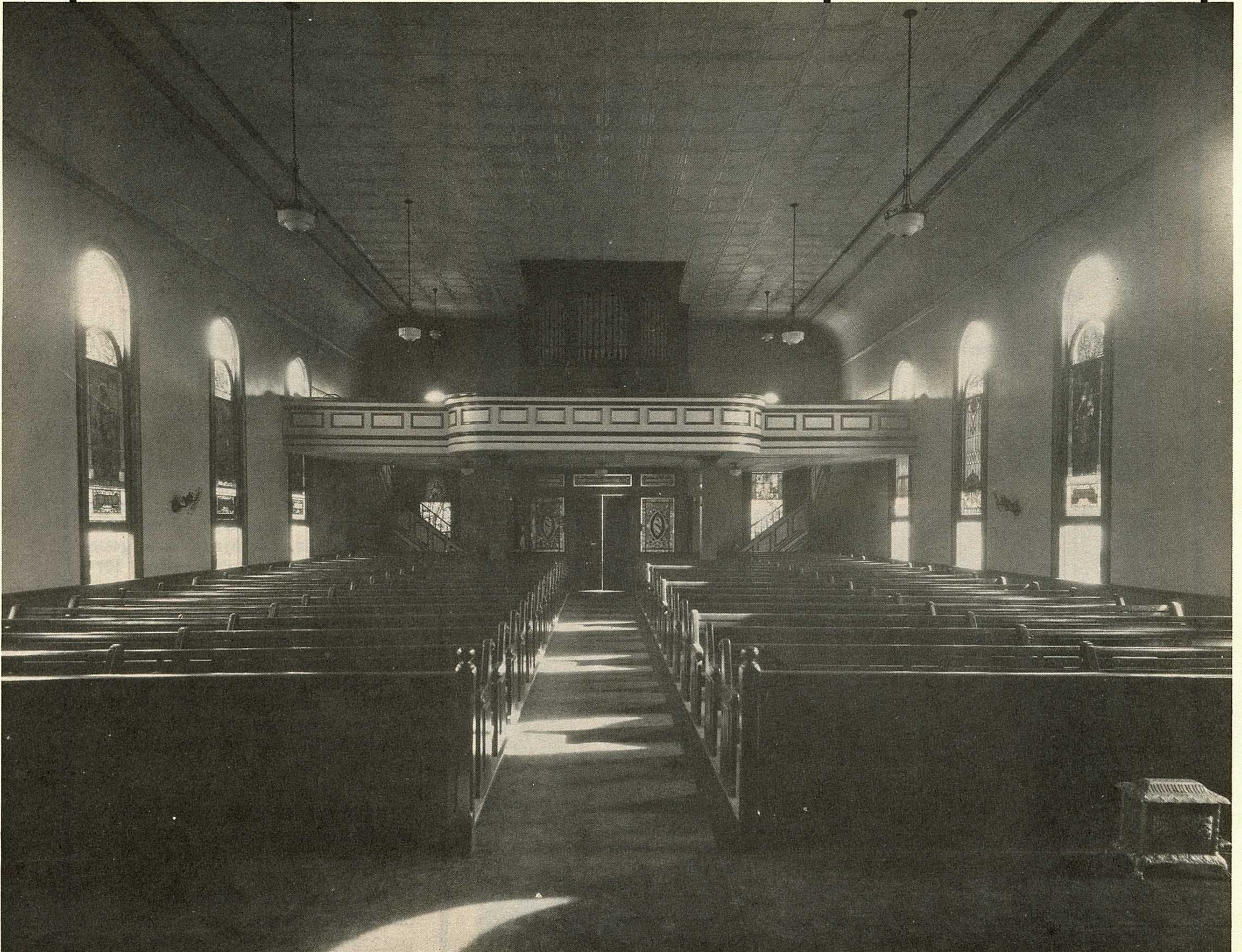
1926 Church interior after the Renovation
