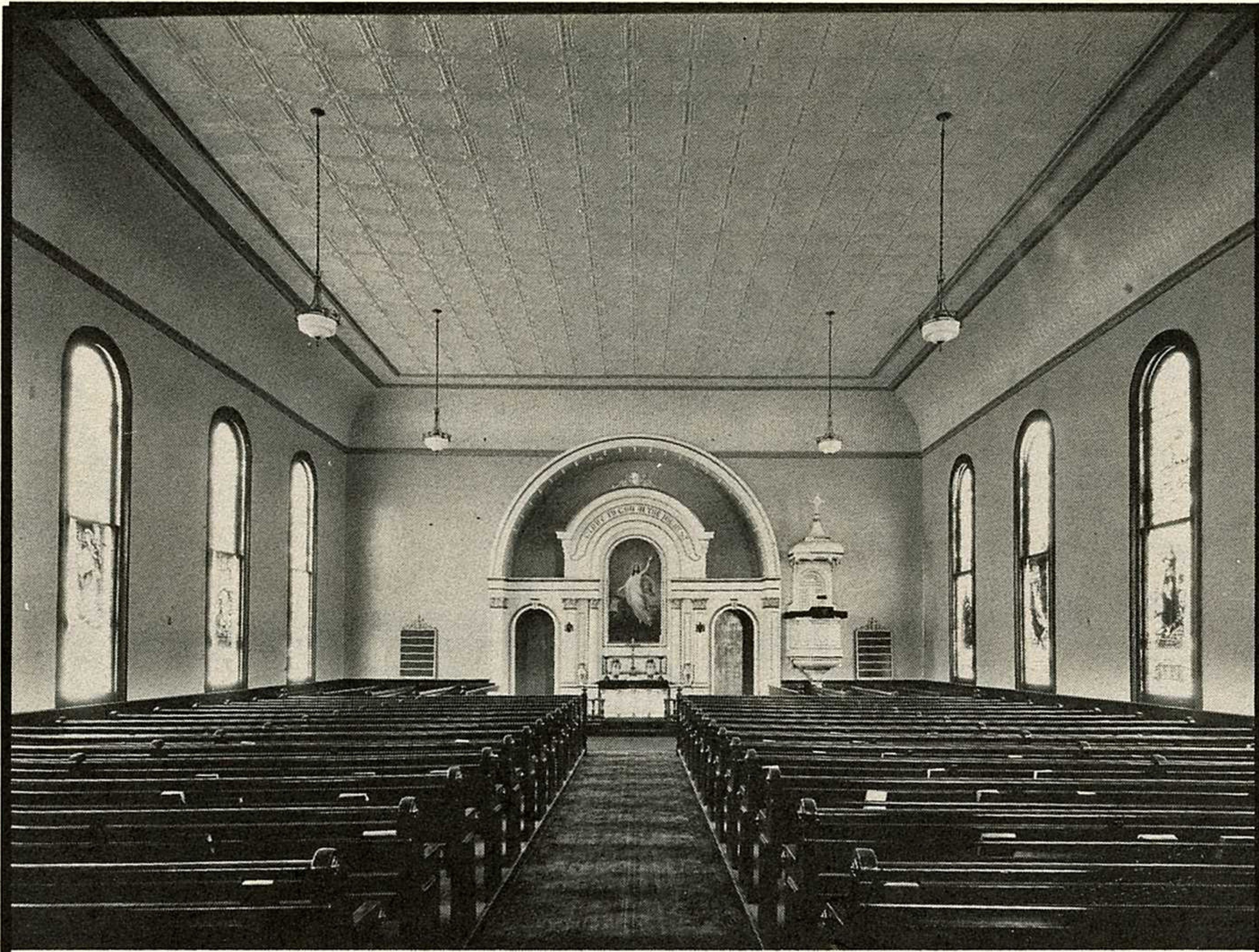
1926 Church interior during the Renovation
